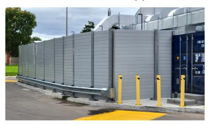
The noise barrier wall was flange-mounted to the curved concrete pad and also supported a curved guardrail.
