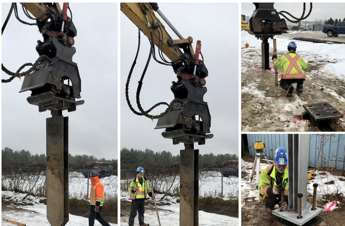
AIL Sound Walls test site for GeoSonic Concrete-Free Foundation Solution
