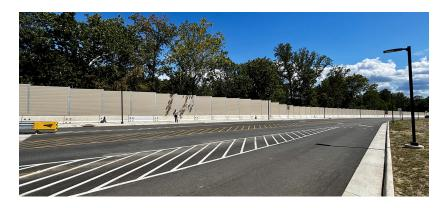
With all this activity, the resort wanted to mitigate the traffic noise along its lengthy entrance road to the complex. The project team selected a Tuf-Barrier (Reflective) from AIL Sound Walls and our lightweight PVC system was able to navigate a number of installation complexities along the 2,067' run.
